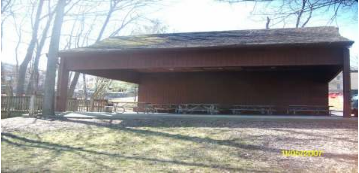
Upper Stage 30ft deep by 40ft wide. 250 South Fourth Street
